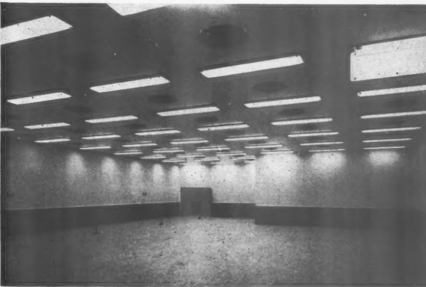
This small factory at Swindon, built by Richard Costain Ltd., is entirely without windows. A completely dust-free interior was required for the production of specialized electrical components, and was the deciding factor in the adoption of this form of design. The artificial lighting inside is at the high level of 85 lumens per sq. ft., which is in line with the conclusions reached in this article.
