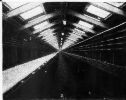
Corrugated 'Perspex' roof lighting at Ince Power Station. It was installed by Cellactite and British Uralite Ltd., sub-contractors to Simon-Carves Ltd. Photograph by courtesy of the Central Electricity Generating Board, North West, Merseyside and North Wales Region.
