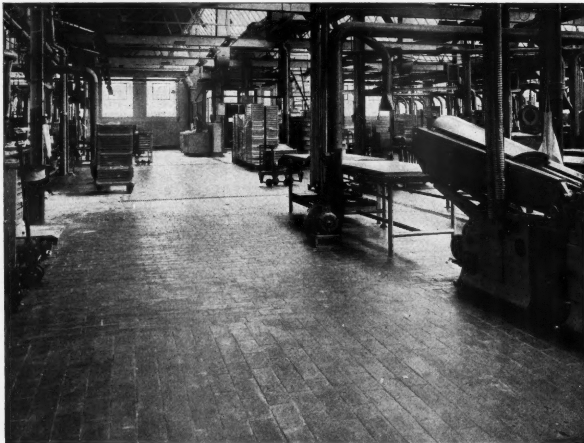
NEW DEPARTMENT FOR JAS. PASCALL LIMITED, MITCHAM 9" x 4½" x 11" Best Red Quarries laid and jointed in special acid and alkali resisting cement Specified by : Gooch & Wagstaff, Chartered Surveyors. Supplied by : Prodorite Ltd.
