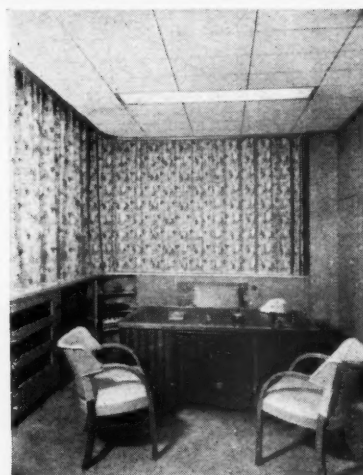
Director's office: Insulated double-wall Compactite partition, veneered and polished light oak. Fittings designed and constructed by Compactom. Acoustic tile ceiling with flush lighting.
