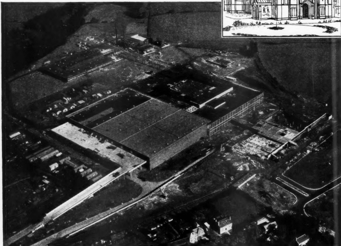
Architect: J. Douglass Mathews & Partners
