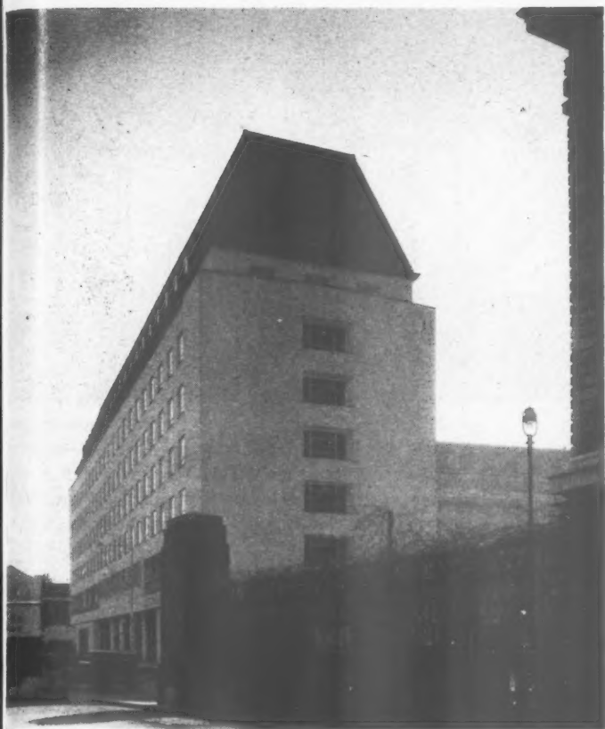
The new LCC building from the direction of the river, showing the solitary central window in the end elevation, which the article claims leaves dark corners inside, and the high flat-topped roof.
