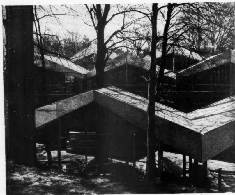
Above: the Swiss pavilion, composed of a series of hexagonal units (steel columns, timber trusses, aluminium curtain walling and cladding). Architect, Werner Gantenbein. Below: the Japanese pavilion, architect Kunio Mayekawa. On the left is part of a traditional Japanese house and on the right is the main pavilion, a steel and glass structure sheltered by a
