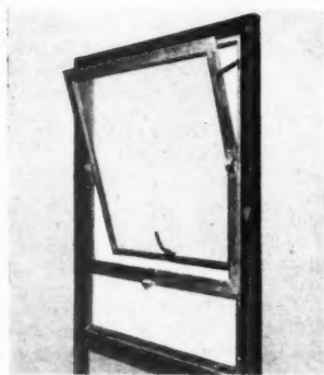
1. Open for ventilation
