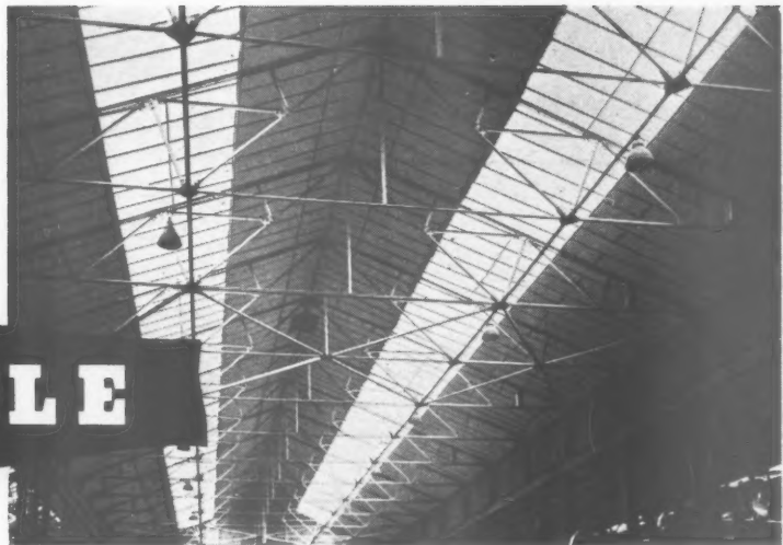
Insulating Gypstele Roof Linings to the Boiler Shop at Messrs. Henry Balfour & Co.'s Durie Foundry, Leven. Erected by Gyproc Products Ltd., Contracts Department
