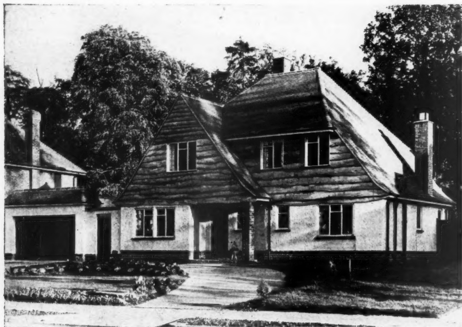
This delightful 3-bedroomed house, the property of Mr. F. A. Holder, is centrally heated by an up-to-date oil-fired warm air system. Shell-Mex and B.P. Ltd. supply the fuel.
