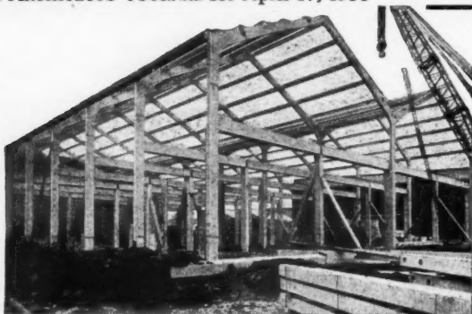
Illustration above shows framework with provision for intermediate floor.
