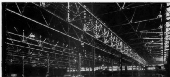
The reinstatement of the fire damaged area in progress of construction.
