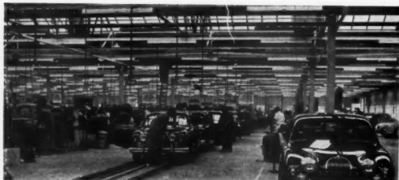
New building erected in 9 weeks.
