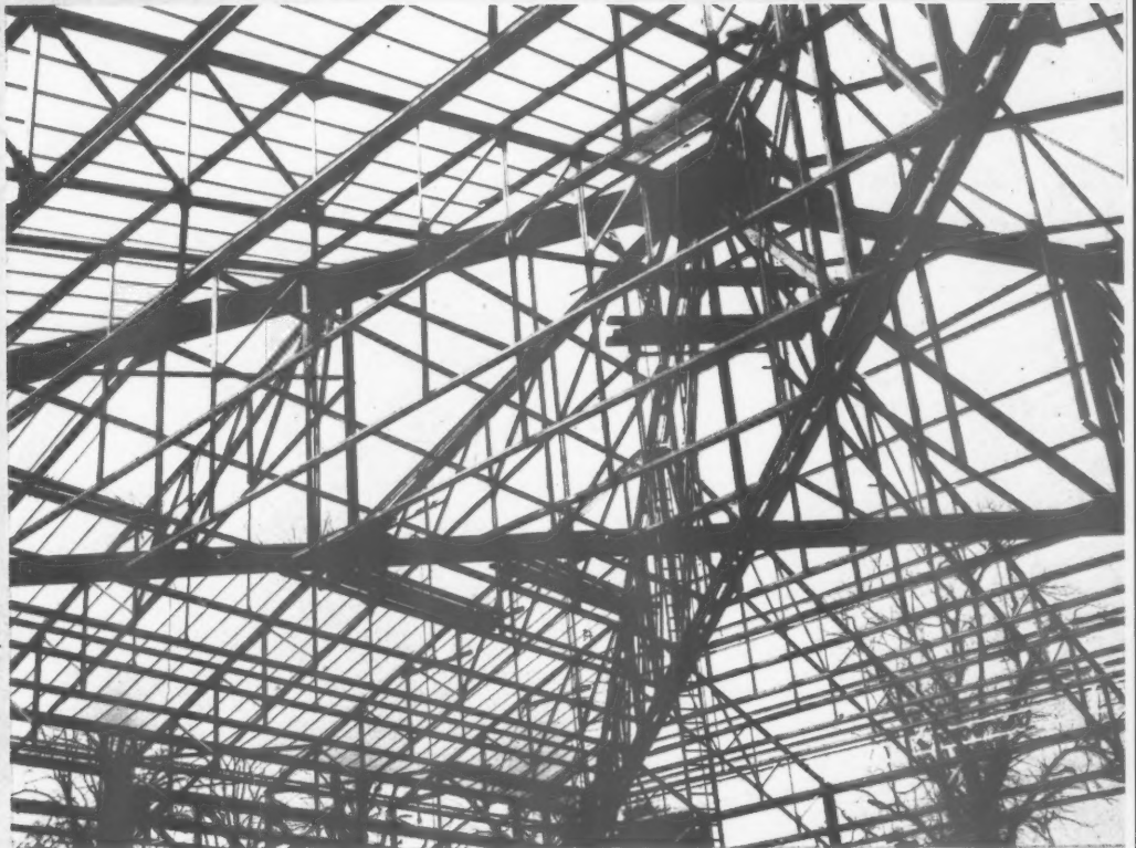
FIXING OF ROOF GLAZING
