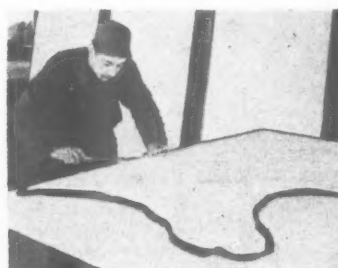
Fig. 11 (below and below centre), detail of American fixing used at Idlewild Airport. The neoprene gaskets are fitted round the panels, the panels are moved into place, and
