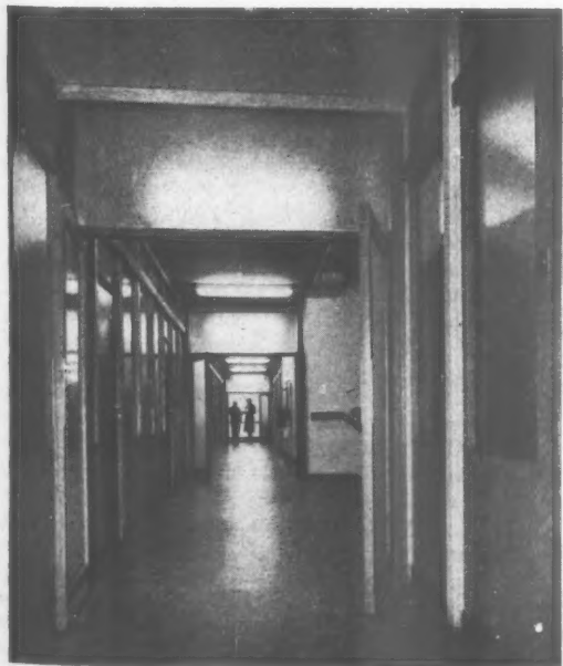
A typical upper floor corridor and staircase landing. Daylight for internal corridors on upper floors is obtained through the glazed office partitions on the east and west sides of the block.
