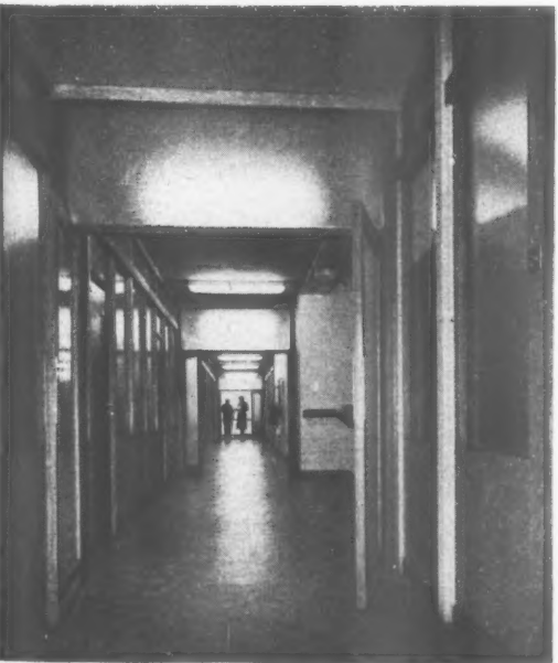
A typical upper floor corridor and staircase landing. Daylights for internal corridors on upper floors is obtained through the glazed office partitions on the east and west sides of the block.
