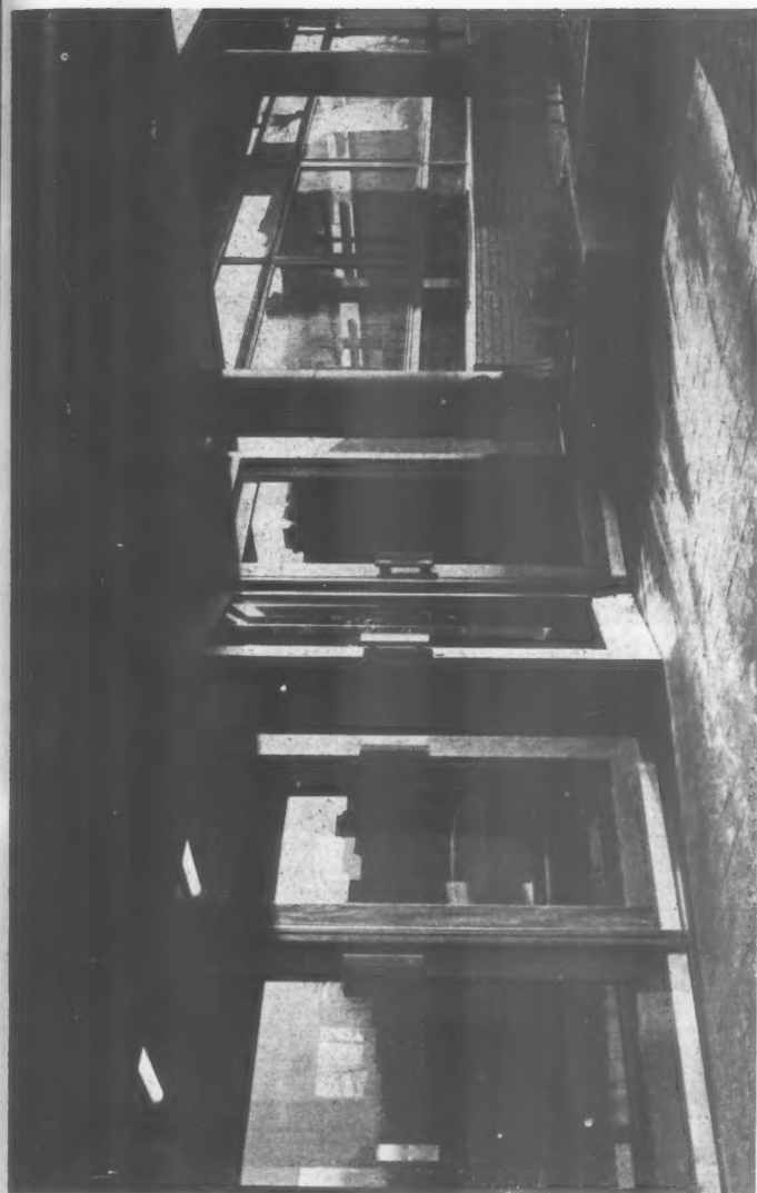
Viewpoint 4 (opposite page, left): the tall staircase window on the east facade and above it the tank and lift motor room. This purpose-made window, which contains fixed and opening lights, is framed in utile hardwood. Viewpoint 5 (opposite page, right): the south facade. Cladding, above first floor level on all facades, is of precast concrete panels with exposed aggregate finish. Windows are framed in hardwood and the 11-in. cavity plinth is faced with Bedford grey-brown bricks. Viewpoint 6 (right): the covered entrance porch. The glazed entrance doors are framed in utile and the flower boxes are of precast concrete.
