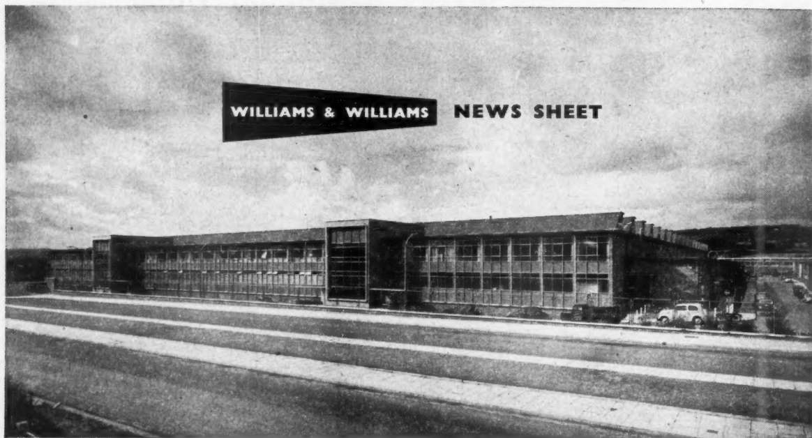
New factory erected by North Western Industrial Estates Ltd., for Mullard Ltd., at Simonstone, Lancashire. Architects: F. J. M. Ormrod, B.Arch., Dip.C.D., F.R.I.B.A., M.T.P.I. and D. H. Mills, B.Arch., A.R.I.B.A., of Ormrod & Partners. Contractors: Holland & Hannen and Cubitts Ltd. Heating & Ventilating Consultants: Hoare, Lea & Partners.
