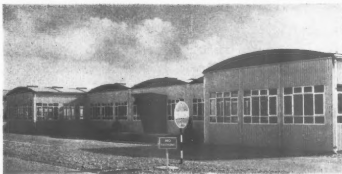
OFFICE BLOCK—10,800 SQ. FT. ERECTED IN 14 DAYS
