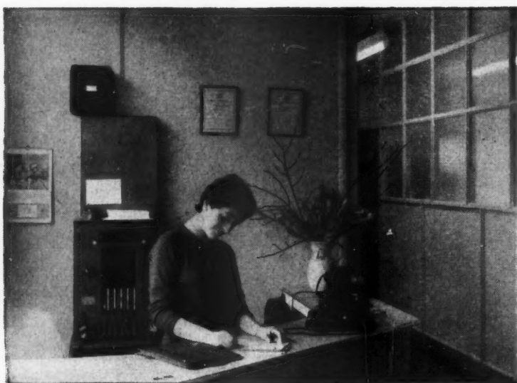
The smart appearance of the office of Max Rayner (Artwork) Ltd. owes much to its new, glazed Stramit partitions in 1-in. x 4-in. timber framing: the Stramit is held in position by quadrant moulds.
