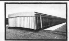
For the new Ford factory at Basildon, Templewood Hawksley supplied aluminium architectural trim and flashings and box gutters of aluminium sheet. The very size of the factory underlines strongly the advantages of using aluminium—no painting necessary, considerable weight-saving, high corrosion resistance, and reduced maintenance.
