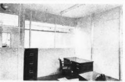
Section of Estimating Office: Half-glazed and full-height partition constructed with Compactite and Tricore panels in aluminium framing.
