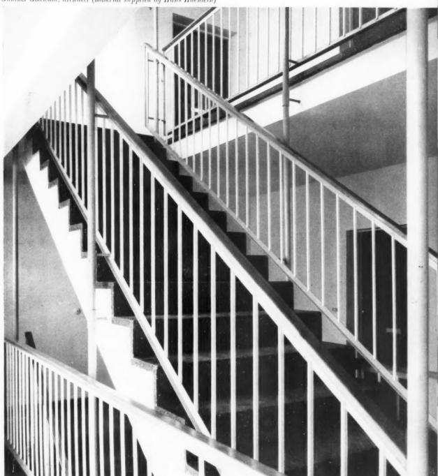
This is a good example of an economical form of stair balustrade. Support for the balustrade is provided by mild steel tubes which rise from the ground floor to the top floor ceiling and which themselves obtain intermediate support from the landing slab. By this means there is no direct connection between the balustrades and floor finishes or stair treads, thus making cleaning easier while at the same time evading an awkward fixing problem. STAIRCASE: FLATS IN BERLIN
