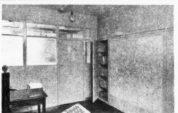
Corner of Wages Office: Hall-glazed Glinex partitions with polished timber framing and Compactom built-in cupboards.
