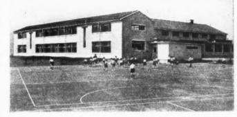
TOPHILL JUNIOR SCHOOL, PORTLAND, DORSET. Architect: J. HURST, A.R.I.B.A., Dorset County Architect. Broderick Insulated Copper Roofing at  $22\frac{1}{2}^{\circ}$  pitch using 28 s.w.g. copper with special fixing to  $2^{\circ}$  Stramit.
