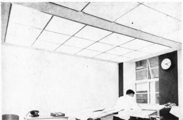
A demonstration installation of the new Lumenator Module lighting system, produced by Lumenated Ceilings Ltd., using plain acrylic plastics diffusers. Some of the decorative vinyl plastics diffusers can be seen at the top of the picture.
