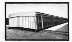
For the new Ford factory at Basildon, Templewood Hawksley supplied aluminium architectural trim and flashings and box gutters of aluminium sheet. The very size of the factory underlines strongly the advantages of using aluminium - no painting necessary, considerable weight-saving, high corrosion resistance, and reduced maintenance.
