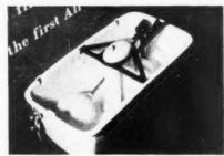
Above left: cut-away of the BRS-developed ball-valve, made by Kings Langley Engineering Co. Ltd. Above right: the Eternum all-polythene cistern by Fordham Pressings Ltd.
