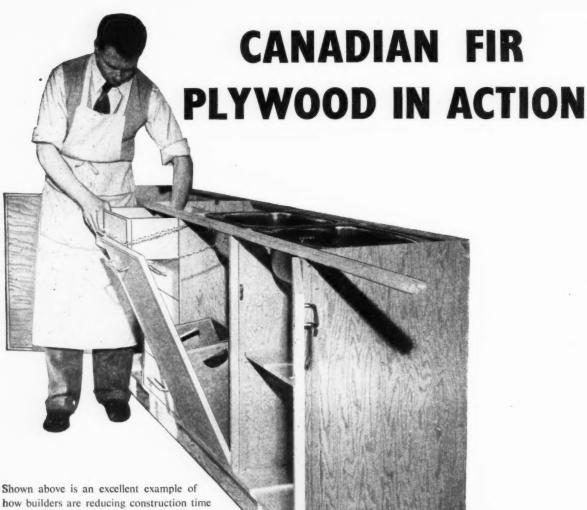
how builders are reducing construction time and getting better results with Canadian fir plywood. This kitchen unit requires little or no framing, yet is strong and rigid. The smooth, one-piece doors are easily cleaned and maintained.
