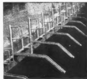
Battery arrangement for bicycles at 12-inch centres.
