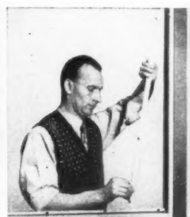
10 Four rubber-buffered glazing beads clip in. Special beads are available for double glazing.
