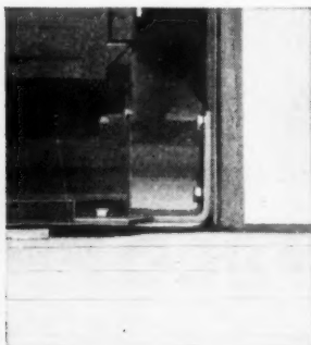
5 The 40" wide modular door frame, linked in with the rest of the system, is firmly anchored at the foot by a cleat.
