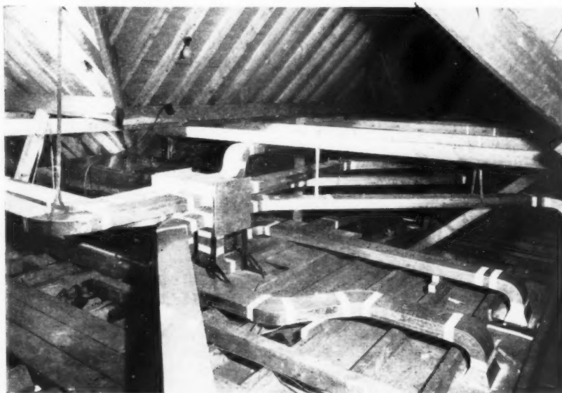
Pak-a-Way heat exchanger unit and duct installed in a roof.
