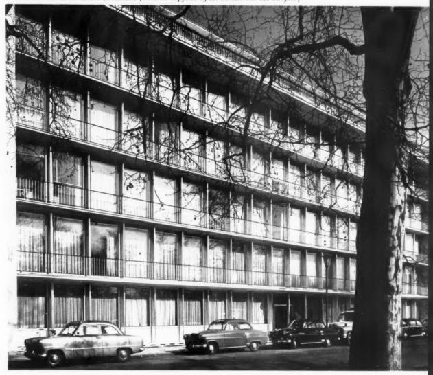
The structure of this facade is unusual in that the main box stanchions are fabricated from two angles welded together and encased in concrete with an anodised aluminium facing.
