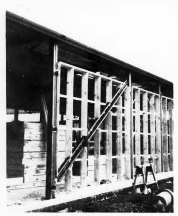
Fig. 9. Prefabricated timber frames for tile cladding. Studs are 1-in. thick planks. Inner linings of \(^3\_8\)-in. thick asbestos fibreboard are fixed to rails and give necessary fire protection. Perimeter stanchions which are always at 6-ft. 8-in. or 10-ft. centres are used universally to support cladding as well as windows.
