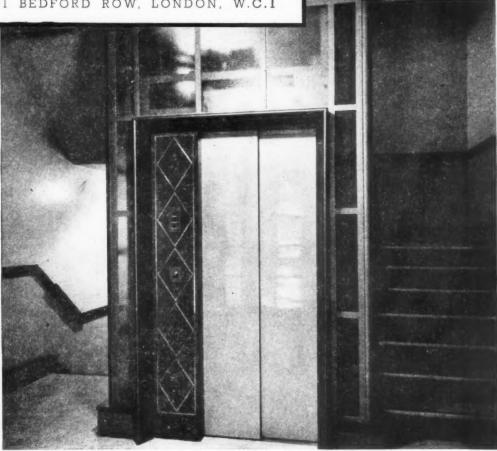
Two seven-person passenger lifts, speed 175 ft. per minute, travelling from basement to 4th floor. Automatic control with automatic return to ground floor. Two-speed - one-way doors.
