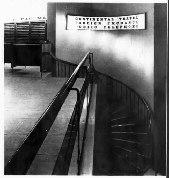
This is a very sophisticated version of the kind of balustrade which has the handrail set several inches on the inward side of the balusters, so that one can lean on it without catching the knees. It was decided to use a mahogany ply handrail as it is a continuation of the stair handrail. The balusters also serve to support a plastic-faced box sign on the balcony fascia.
