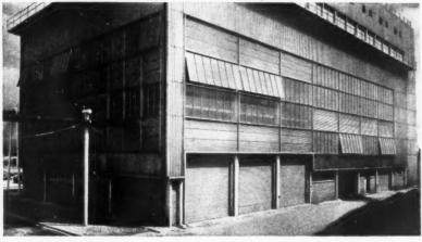
The interior of the compressor house showing the runs of Aluminex' sidewall glazing under the caves and the gear-operated vertically pivoted aluminium windows. The gable end is clad with 'Wallspan'. A feature of this building is the way in which possible gas traps in the roof have been avoided by omitting a central ridge. The highest point in each bay is occupied by opening windows designed to give maximum ventilation.
