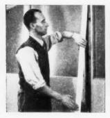
8 Pilasters are clipped on to the finish off the joins between units.
