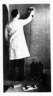
Above, washing a wall down with the Revvi equipment. One of the cylinders contains detergent, the other, rinsing water. Several shapes of pad are available. Right the Rayburn No. 2 boiler.
