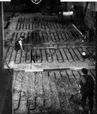
Photograph shows typical installation of coils for floor panel warming system.
