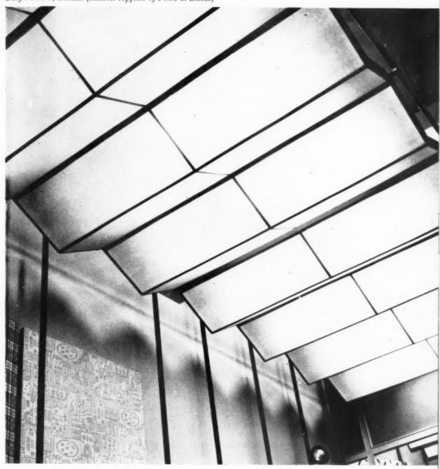
The false ceiling was introduced to lessen the height of the small room and provide an economical diffusion of light. It shows an original use of common materials.
