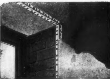
Protection of a window reveal.
