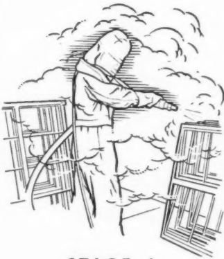
STAGE 1 Preparing the surface
