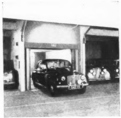
Above, a car leaving the lift and running on to the distributing trolley (see plan below) at the vertical car parking garage designed by William Wadsworth & Sons Ltd.
