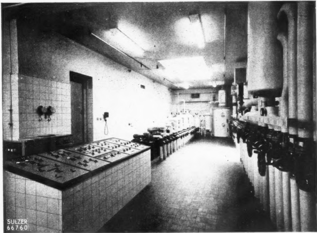
Hot water valve and collecting equipment in a heat supply station.
