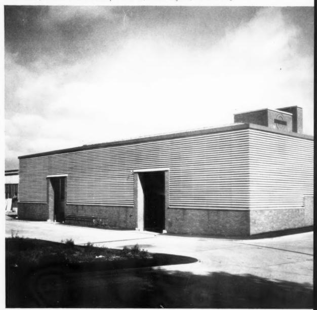
Asbestos touvre blades have been used instead of wood to save maintenance and because there was no serious danger of shattering. The neat appearance is largely due to the fact that all fixing is concealed from the outside.
