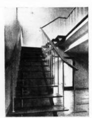
Stairway in hall outside the linear accelerator room. The wooden treads are supported on 3/16th-m.s. sheet angles from the 6-in. × 2-in. stringers. The timber for handrails, stringers and treads is sapele.
