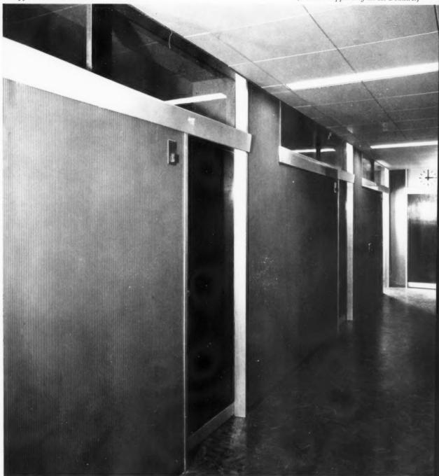
The interest of this detail lies in the finishes, which are typical of new office buildings in Milan. The partition is of rendered clay blocks to which a ribbed grey linoleum has been stuck. Apart from the sill (which is hardwood painted bright yellow) all trim is formed of anodised aluminium extrusions. The door is solid-core timber, faced with a plain linoleum coloured deep blue-grey.
