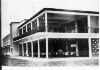
ventilation throughout the building. This is essential in the humid-tropical atmosphere of Malaya. On the entrance side (top) exterior walls and windows were dispensed with in favour of aluminium adjustable sun breakers (seen extreme left, above). These are hand-operated and are adjustable through 180°. Because of their interlocking nature, they resist rain and yet provide necessary ventilation. Left, on the elevation facing the runway aluminium projected "push out" windows were
