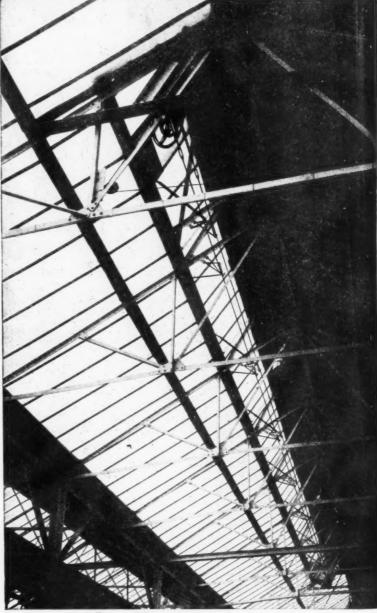
The illustration shows One set of Electrically operated Twin Tension Koo Gear with Countries Balance Unit operating one continuous opening light, 74' 0" long × 5' 0" deep. Note the Spiral Bal nce Wheel fitted at the end sprocket
