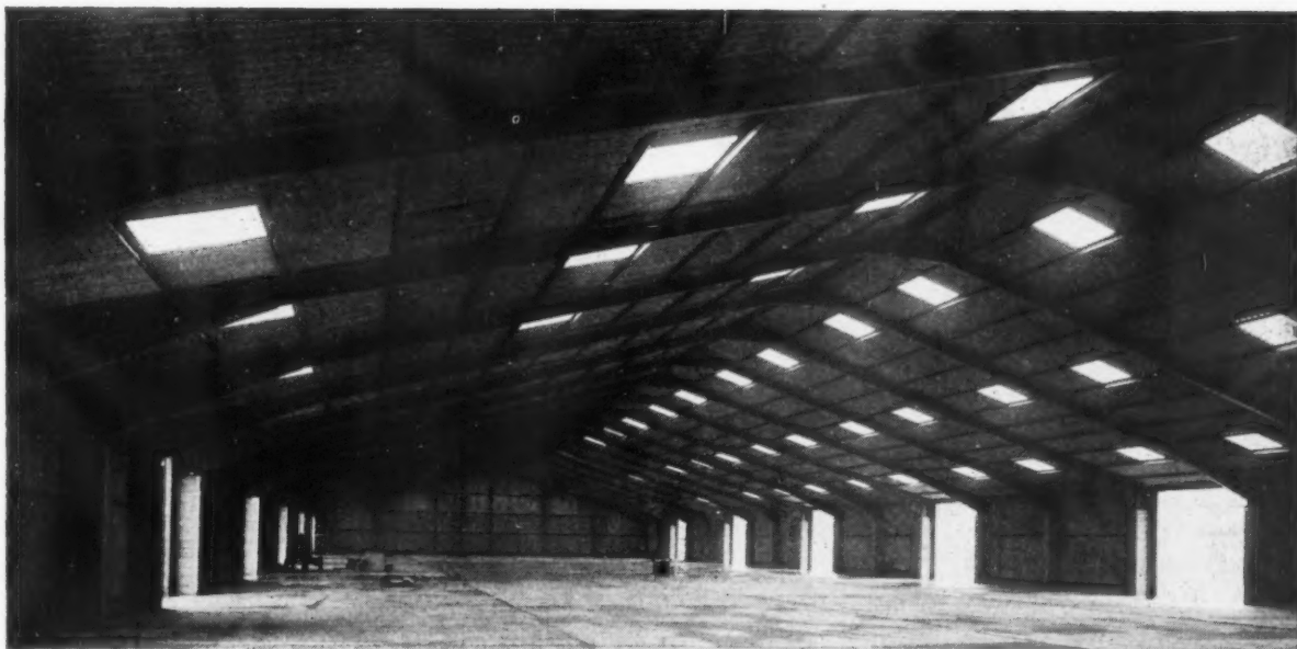
Warehouse Length 300 ft. Span 101 ft. - 6 ins. Pitch 17° Architects: Fowler Grove & Haggar Southampton.
