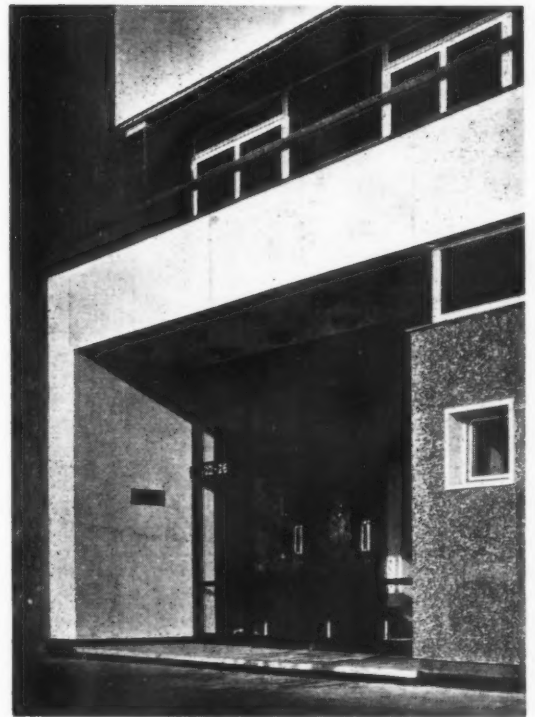
Viewpoint 4: the main entrance. The metal door and frame is painted black. The pre-cast terrazzo and reconstructed stone slabs are cramped back to in situ concrete or brickwork behind. The asphalt tanking of the basement is brought a few inches above ground level to form a plinth on the face of the building.
