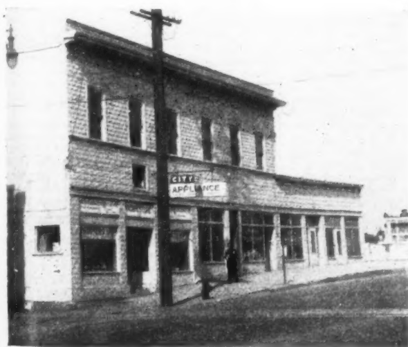
W. W. Ryder writes above about prefabricated (steel) stonework in Switzerland. Here is a photograph of the same sort of thing in Wisconsin, which a New York correspondent mentioned in our issue of September 6.
