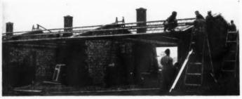
Fig. 7 (top left): the completed dwellings on the Coldharbour estate at Woolwich. Fig. 8 (above left): during construction, showing the load-bearing cross walls and lattice roof joists. Roof support at the eaves schedule, £258 wages of a costing clerk, and exceptional time spent on supervision and costings, £21 for sundry development labour, and £64 expenditure on technical and press visits and the opening ceremony.
