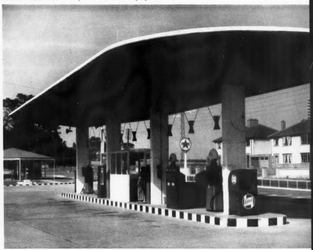
The roof of the canopy is stiffened by tapered upstand beams running from the outer rim inwards to an upstand spine which spans between the columns. Rainwater is carried off the roof by copper r.w.p.'s running through the centres of the columns.
