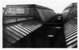
Viewpoint 10: typical junction of high and low level monitor roof lights. Those in the centre of the building have patent glazing at an angle of 61 degrees, flanked to north and south by patent glazing at 39 degrees. The roof finish is asphalt on 3½-in, thick r.c. slabs.
