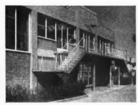
Above (viewpoint 9): the external staircases at the south-east corner of the building, leading to the workers' canteen and lunch room on the first floor. External walling consists of 9-in. mass concrete on the ground floor, and two skins of 6-in. concrete blocks, with cavity, under first floor windows. The stairs are of r.c. construction.
