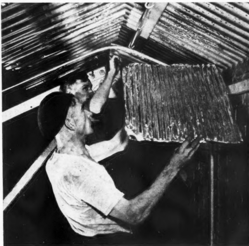
Fixing corrugated sheets of Venesta aluminium foil in position.
