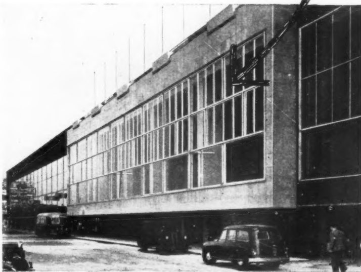
Windows by Williams & Williams Ltd., using Timinium alloy, at London Airport. Architect: Frederick Gibberd
