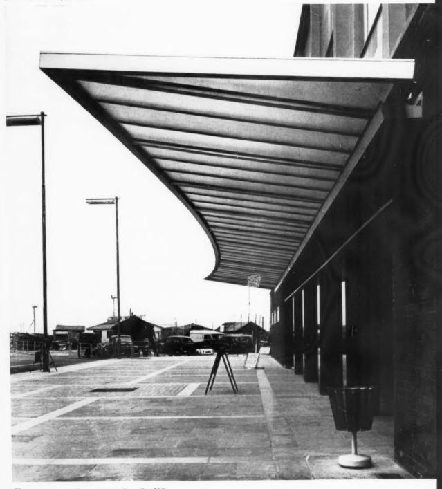
The canopy is supported on purpose-made r.s.j's which taper along their length and, passing over the top flange of one r.s. beam directly behind the wall face, are botted to the web of another 6 ft. further back. The fascia is formed in aluminium-faced plywood clipped to a r.s. angle and the same material is used to box in the supporting r.s.j's.
