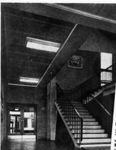
The National Coal Board Laboratories, Cheltenham, are always comfortably warm and delightfully quiet—thanks to Frenger Ceilings. Frenger is a heated acoustic ceiling made up of a pipe grid (connected to the hot water heating system) supporting perforated metal panels and blanketed by insulating material.
