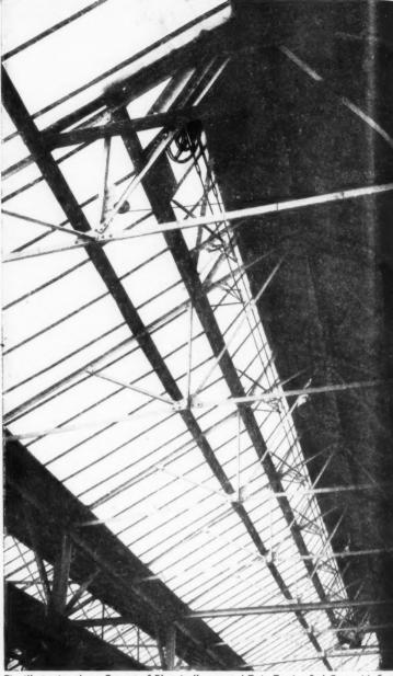
The illustration shows One set of Electrically operated Twin Tension Rod Gear with County Balance Unit operating one continuous opening light,  $74^{\prime}$  0 $^{\prime\prime}$  long  $\times$  5 $^{\prime}$ 0 $^{\prime\prime}$  deep. Note the Spiral Balance Wheel fitted at the end sprocket.
