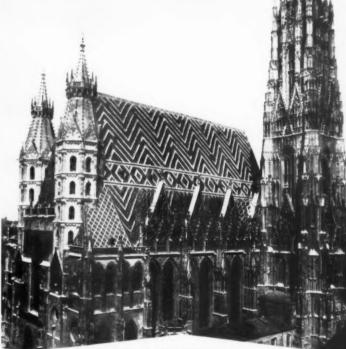
YLAMON IN A PREVENTATIVE ROLE After the war, the roof of St. Stephen's Cathedral in Vienna had to be completely rebuilt. Preservative treatment was essential. It was carried out quickly and economically on site by dipping the timber in large open troughs prior to erection. 700 gallons of Xylamon were used.
