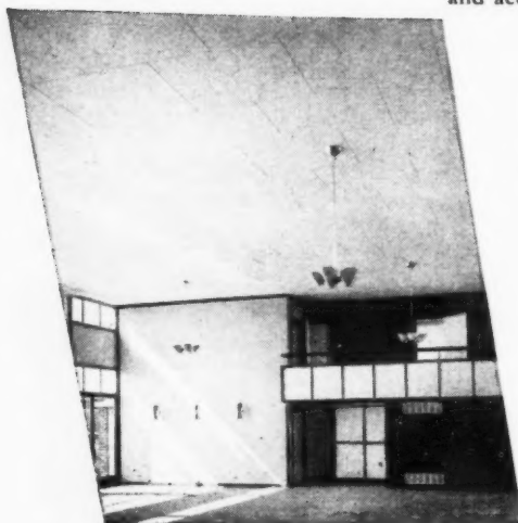
Suspended ceiling of ASBESTOLUX at the Peter Lea County Primary School, Fairwater, Cardiff.
