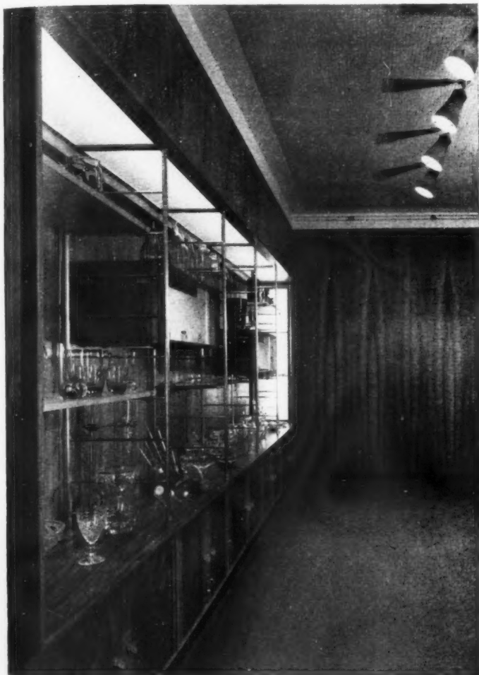
Fig. 7: an example of the application of veneering to wall panelling and to fitments. The whole of these veneers are here applied to one of the chipboards which has been used both for the panelling and in the construction of the fitments.
