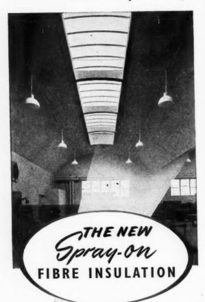
Because of its barrel-vault construction, the roof of the new B.T.C Apprentices Training School at Crewe demanded the spray technique of insulation, and a one-inch layer of Asbestospray—the new sprayed fibre which can be applied to any surface—was applied by Kenyon's, the sole contractors. In addition to remarkable acoustic and thermal insulation properties, Asbest spray is extremely light, economical and decorative. For full details write for leaflet.
