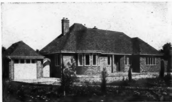
Private Residence at Hexwall.
