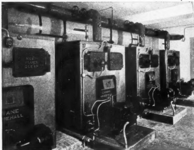
These four No. 410.L. Whitehall Sectional Heating Boilers are each rated at 936,000 B.Th.U's per hour.
