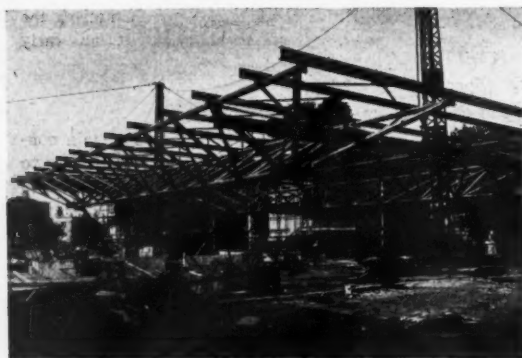
Left: assembly hall roof of the Mayfield School, Putney. Architects, Powell and Moya; engineer, Ove Arup and Partners; structural contractors, Carter Horsley Ltd. The 27-ton space frame was fixed together on the ground and hoisted in one piece, before the stanchions were erected. This is one example of the advanced methods of which some contractors are now capable. Above right: LCC point block at Trinity Road, Wandsworth (Architect to the Council, Dr. J. L. Martin; engineer, Ove Arup and Partners). The contractors, Wates Ltd., devised the suspended cradle which started from ground level with bricklayers building the external walls, and then descended from the top for external painting and glazing. In wet weather a roof is put on the cradle.
