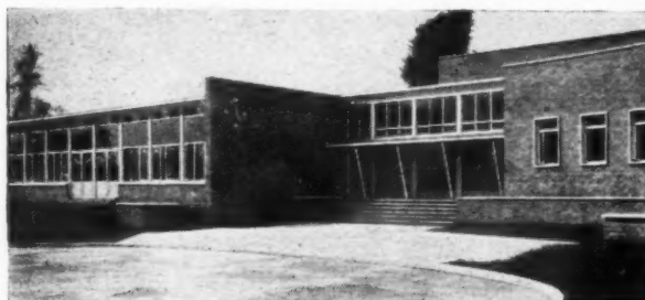
A main entrance and classroom block
