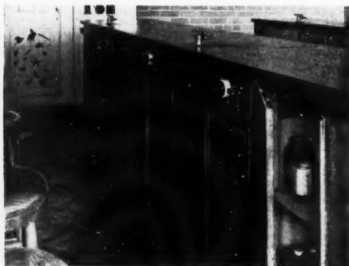
Science benches which are fitted with gas and low-voltage electricity (from batteries on right). Upper floor plumbing is simplified by not fitting sinks into island benches.
