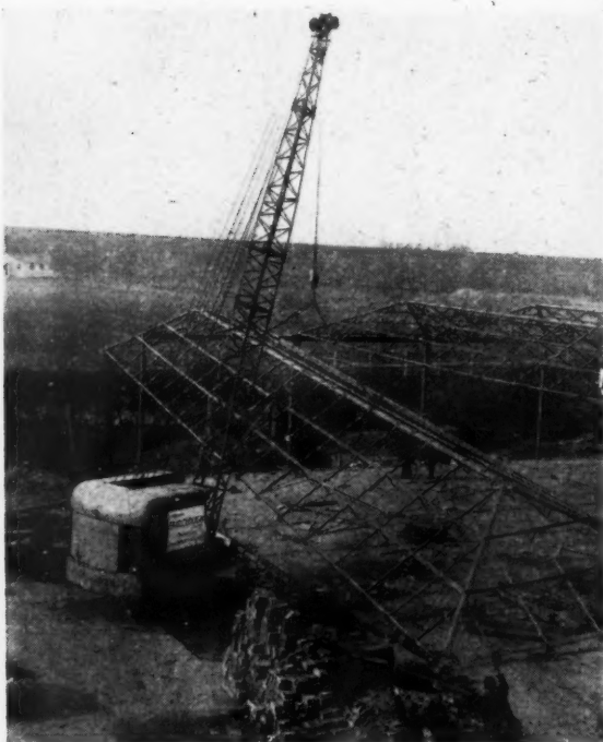
90ft. clear span pre-stressed steel frames assembled on the ground are lifted into position. Consulting Engineer: F. J. Samuely, B.Sc., A.M.I.C.E., M.I.Struct.E.
