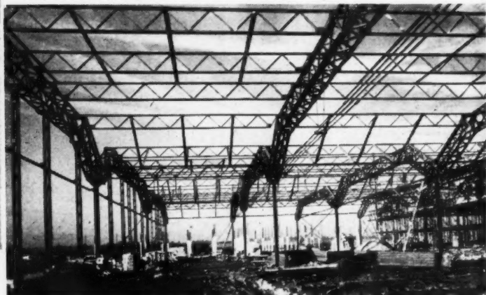
Pre-stressed steelwork of a factory for occupation by Standard Telephones and Cables Ltd., built by Harlow Development Corporation. Frederick Gibberd, F.R.I.B.A., Architect Planner to Harlow Development Corporation. Structural design by R. A. Sefton Jenkins, B.Sc., A.C.G.I., A.M.I.Str.E., A.M.I.C.E.
