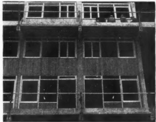
Fig. 12 (left). Details of external panels on access balcony side of 11-storey block. Fig. 13 (above). External panels on private balcony side of 11-storey block.
