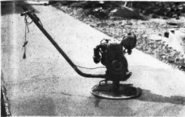
Fig. 3.—A power float with rotating disc which is claimed to do the work of eight plasterers, and which requires a lower water/cement ratio. The screed can be walked over immediately after floating. Photo: M.O.W. Crown copyright.
