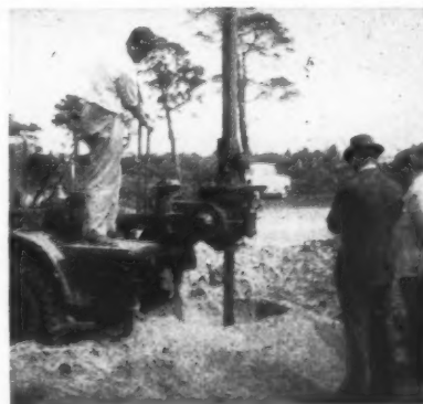
Fig. 6. Mobile borer for short bored piles on shrinkable clay sites. The latest types under-ream the borehole providing an expanded foot on the pile.
