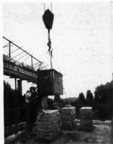
Fig. 2.—Moving bricks in quantity. The box is detached from the pallet to go back for the next pallet-load.
