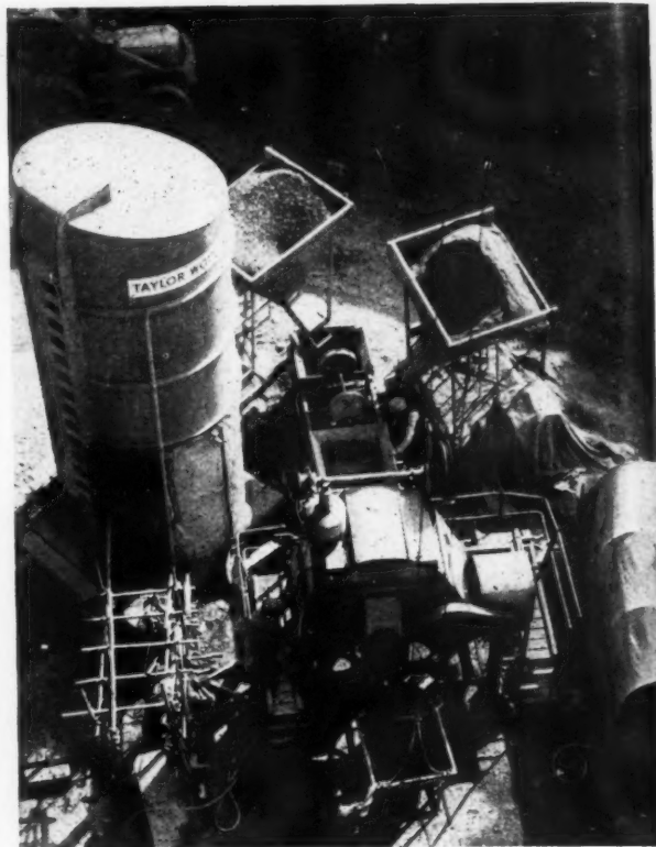
Fig. 1.—Concreting plant with 21/14 mixer, 20-ton bulk cement silo and double swing weigh batcher. The hoppers are fed by the loading tractor in the background. The \frac{3}{4} cubic yard bottom and side outlet skip (being filled) takes the full batch of concrete and is hoisted by the tower crane to the placing point.
