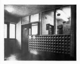
The photograph, left, shows the entrance hall of the two-storey office block. The panel below the enquiry window is of glazed tiles in yellow, black, grey and white. The floor finish throughout the ground floor is thermoplastic tiling. The office block contains a showroom for finished products, a drawing office, general and managerial offices, cloakrooms and lavatories.
