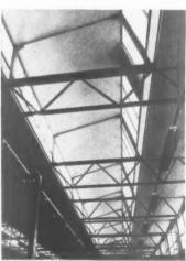
Above left, section through the end bay of the production area adjoining the works offices. [Scale:  $\mathbf{i}'' = \mathbf{i}' \mathbf{0}''$ ] Above right, view of the end bay, showing the secondary lattice beams. These are supported on 7-in. by 4-in. stanchions at the perimeter, and 16-in. by 6-in. primary beams internally.
