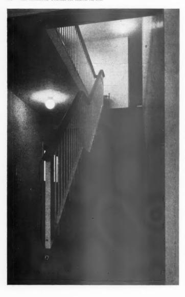
Left, the staircase in the two-storey office block. The treads are finished with granolithic concrete. The walls to the offices and circulation areas are white, colour being used only in small areas, such as the doors, which are yellow-green. The landing at the top of the staircase is lit by clerestory windows looking out over the roof of the production area. An alternative means of escape in case of fire has been provided by a steel ladder from the first floor to the production area.
