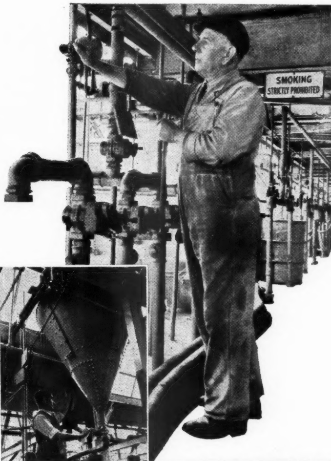
Calibrated cones for measuring solvent supplies.
