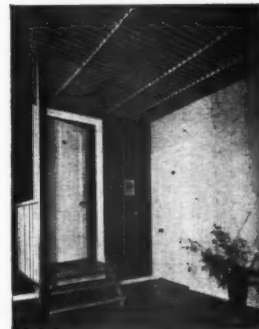
Left, the reconstructed first floor landing with suspended ceiling to camouflage the excessive ceiling height. Right a typical bedroom arrangement
