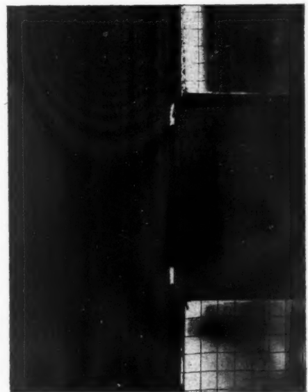
A joint between the stile and rail of a glazed door, which has opened up through moisture movement. The door was fixed some time before the heating in the building was turned on, and the shrinkage was accentuated by the fact that the stile was a very wide one.
