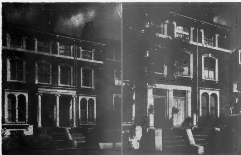
Local Authority improvements in Cambrian Road, Richmond. This crude approach to cutting maintenance and repair costs by slicing off porches (right) isn't good enough. It spoils the whole street character and mutilates the proportions of the individual elevation. These houses can be assumed to stand for at least another half century. Such a massacre should be strongly discouraged.
