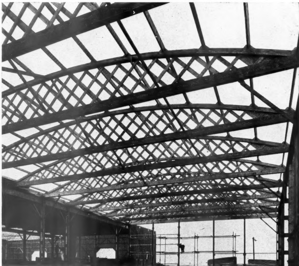
Laminated timber trusses of 60 ft. clear span in the Company's new storage shed at Tyne Dock, Newcastle
