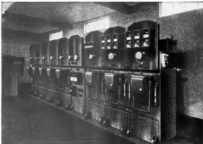
"Ellison" 11,000 volt switchboard in a factory of the Gloster Aircraft Co.
