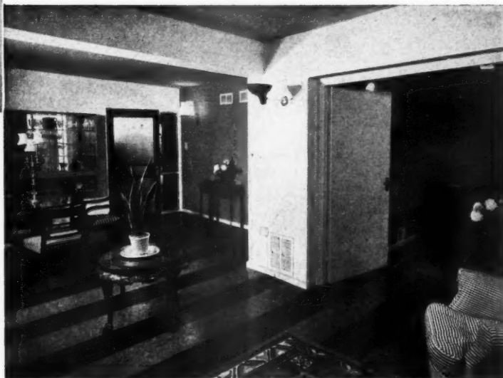
Warm air inlet register and high level return air grille, unobtrusive yet effective. The room thermostat controls temperature.
