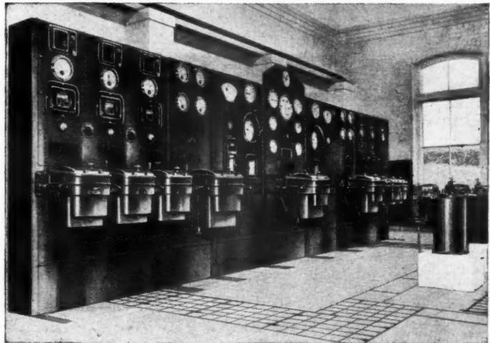
"Ellison" 400 volt switchgear in a Pumping Station of the Cheltenham and Gloucester Water Board.
