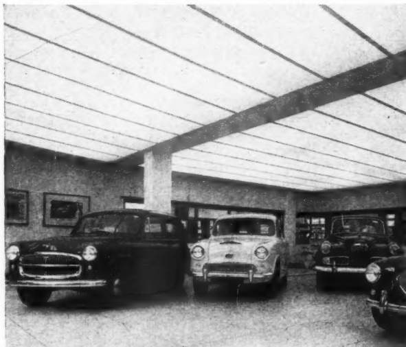
Above and right: the Lumenated ceiling. Flexible translucent plastic sheets fixed between m.s. H sections 3 ft. apart.
