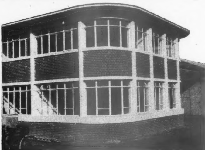
New Office Block for Messrs. Leonard Stace Ltd., Cheltenham: Architects: Messrs. Ellery Anderson, Roiser and Falconer, L/A.R.I.B.A. (The framing, first floor, roof, and canopy all in reinforced concrete by Homan and Rodgers Ltd.)
