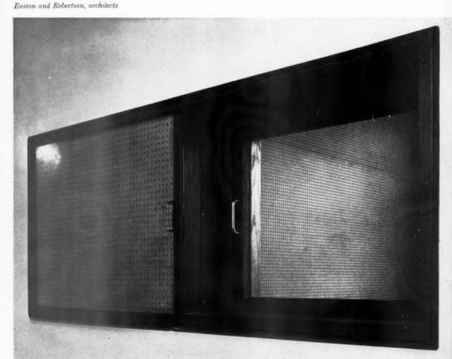
This observation window forms part of the heavily soundinsulated construction of the audiometry room. As the room is for testing the hearing of children, the inner window (i.e. that farthest from the camera) is built up from two sheets of glass with a transparent silvered surface between, so arranged that observers can watch the children without being seen by them. OBSERVATION WINDOW, AUDIOMETRY ROOM: HOSPITAL IN LONDON, W.C.1
