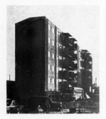
Fig. 1. General view showing the flats nearing completion. The balconies are constructed of precast concrete slabs supported on a framework of  $2\frac{1}{2}$ -in. dia. steel tubes.
