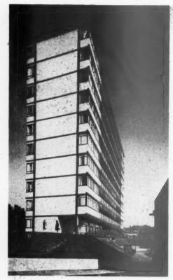
Above; the south-east and north-east facades of the block of flats. The exposed concrete frame is painted dark red and light grey. The bricks are white flint limes.
