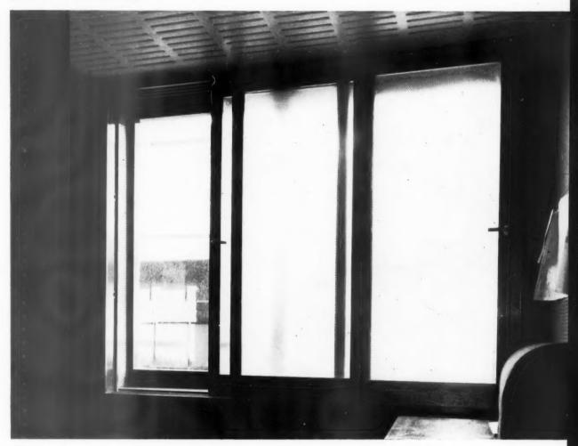
The window and door to the audiometry room are both of double construction. Each door panel consists of two skins of acoustic board with slag wool between, veneered on the outer side of the door with teak.
