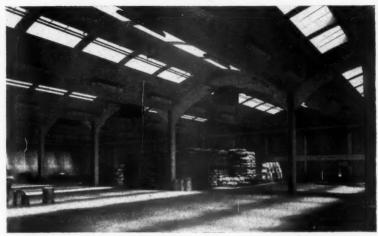
a barrel vault roof to the production area, and r.c. columns, floor and roof slabs to the office block. The ground is shrinkable clay, generally fairly firm, but as numerous pockets of softer clay were encountered the majority of the 61 bases to the columns were individually designed to suit the exact site conditions. The 4-in. blinding concrete was laid direct on the dry clay immediately the levels had been reduced, with holes left for excavating
