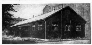
For sectional timber buildings consult Hall's. Hall's standard 6 ft. unit can be assembled to any length in spans of 10 ft., 12 ft., 15 ft., 18 ft., 24 ft. and 30 ft. Built throughout of selected, fully seasoned timber (Hall's have their own timber drying kilns) they are widely used as Classrooms, Village Halls, Community Centres, Recreation Rooms, Canteens, Factory extensions, etc. Fully detailed plans supplied against your specification.
