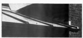
Detail of roll cap roof at eaves.
