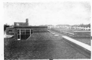
PERMANITE WOODWOOL INSULATED BUILT-UP FELT ROOFING is adaptable to all types of roof plan. It is economical in construction and quickly laid by our own expert craftsmen.
