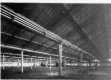
Above right, aerial view of the factory from the north-west. Above, part of the production area of 300 ft. by 240 ft. Left, another view of some of the 30-ft. sq. bays in the production area. The frames are of welded steel.
