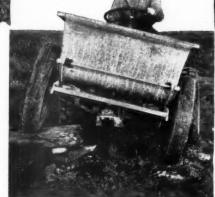
The Floating Front Axle allows either wheel to mount a 16" obstacle.
