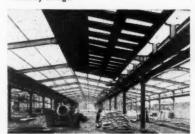
Multi-span all welded Construction
