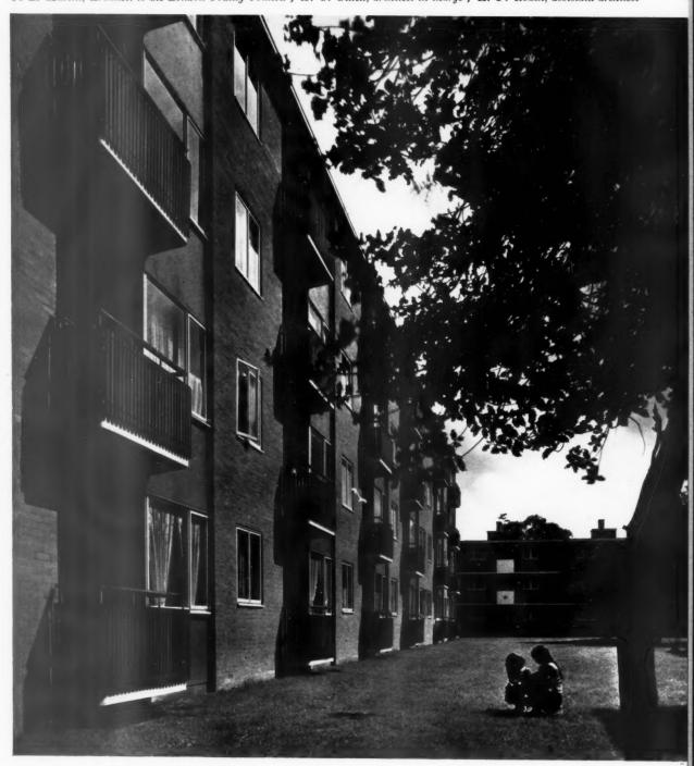
The balcony framing, comprising the uprights, the core to receive the handrail and the horizontals to receive the hardwood slats, was prefabricated in one piece. As this framing is sufficiently secured to the in-situ concrete floor it has no point of junction with the brick.
