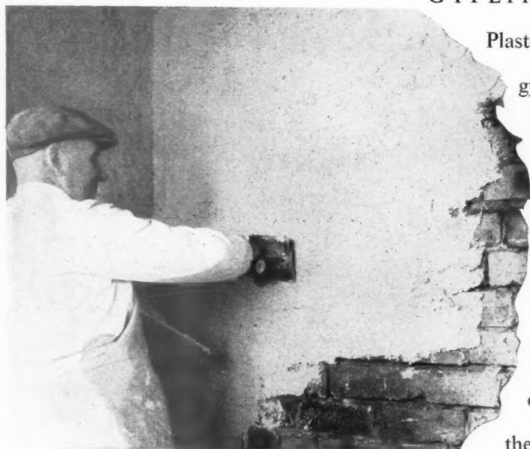
GYPLITE Undercoat Plaster being applied over brickwork in the usual manner.
