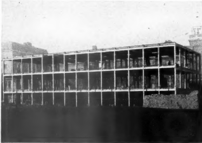
Above: Front elevation showing framework of multi-storey precast structural units.
