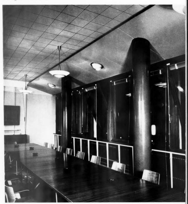
The purpose of the sloping baffle is to direct smoke and used air, rising in the centre of the room, outward to the louvres. Should natural ventilation prove insufficient, allowance has been made for the fitting of an extract fun.
