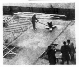
Fig. 11, a floor screed being finished and polished by machine. The near floor slab is already finished, the further slab, with heating panel laid, awaits its screed.
