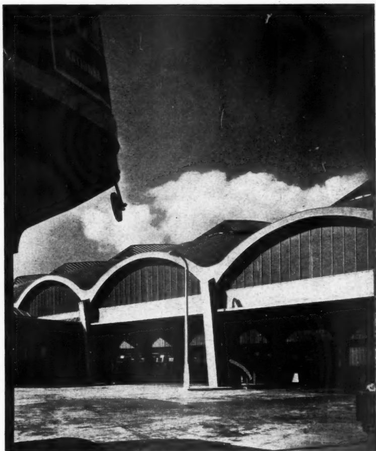
PLAN. —The main influence on the design was the need for unrestricted floor space to accommodate the requisite number of vehicles. On this irregularly-shaped site the parking area had to be situated at the largest end—the north end. The offices and staff rooms are contained in a separate block on the Bin-
