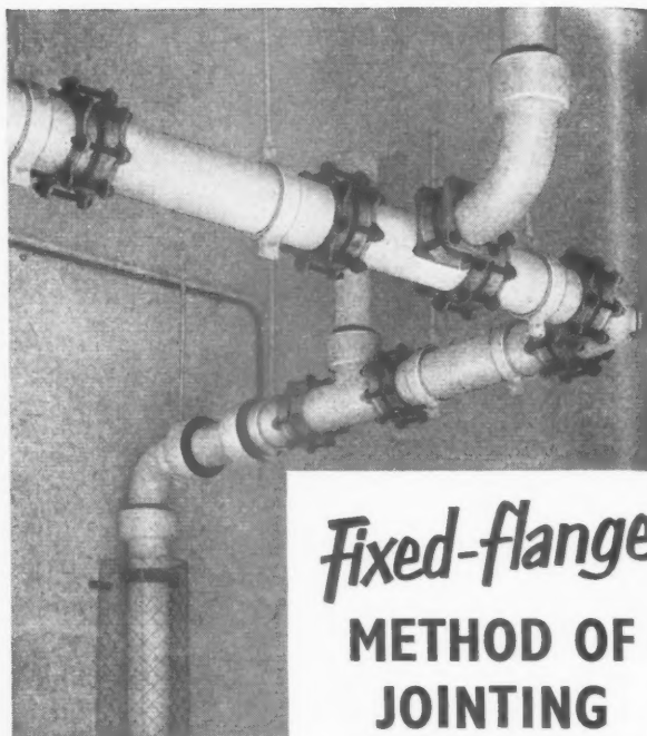
Royal Doulton acid proof white chemical stoneware pipe lines at the Imperial College of Science & Technology, South Kensington, showing the fixed flange method of jointing.
