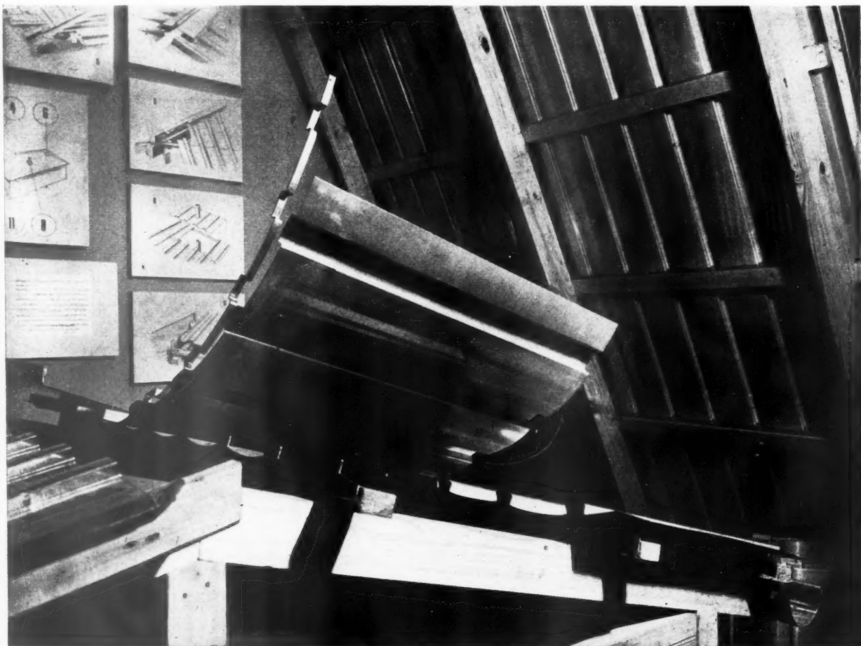
A mock-up of part of a "Fural" roof which was on view at Olympia. On the right is a typical underside of a "Fural" roof. Note the very clean appearance.
