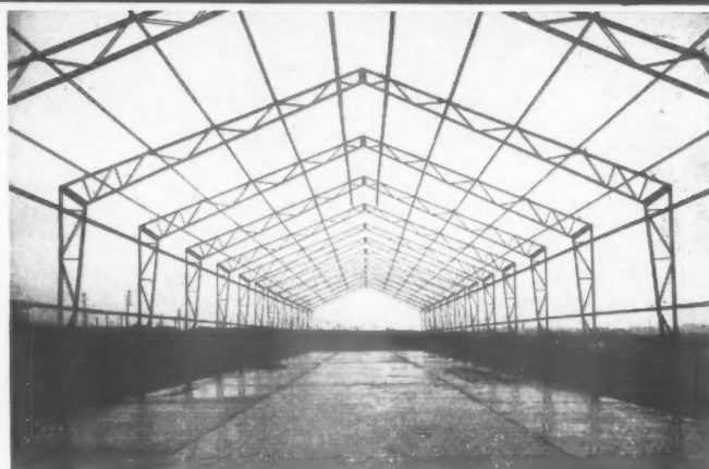
Large sliding Doors Perspex Roof Lights or Patent Glazing. Steel Framed Windows. Completely or partly clad in Asbestos Cement.
