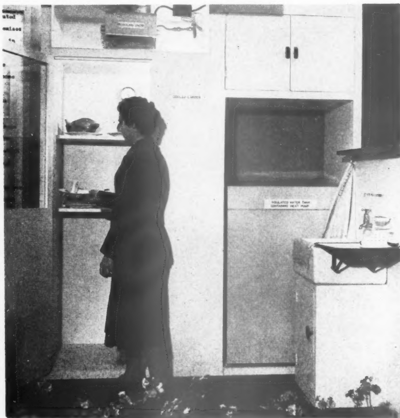
Domestic heat pump installation, providing space heating, domestic hot water and cooling for larder. The cooling unit can be seen top left; the pump is in the insulated water tank, behind the sink. See note below, right.
