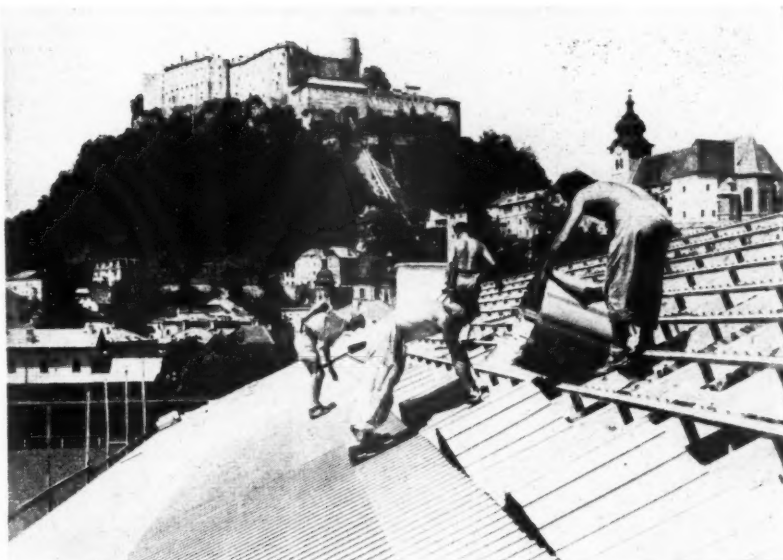
Above, workmen laying a "Fural" roof at Salzburg. Rubber-soled shoes are recommended. The sheets are unrolled and temporarily clipped into position, leaving enough play for the roofer to bend back the sheet in order to open up the ribs as he works along.
