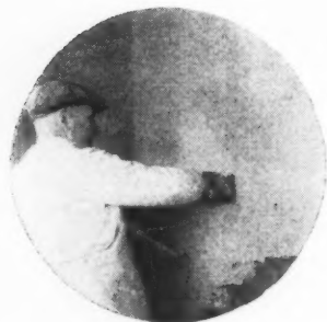
GYPLITE Undercoat Plaster being applied over brickwork in the usual manner.
