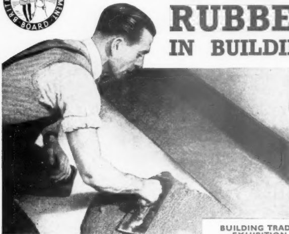
Floor being surfaced with latex/cement composition.
